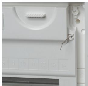
Sealing holes to protect against unauthorized access.
