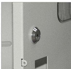
Operational panel covering the electricity meter and electrical devices. The panel is attached to the enclosure with hinges and locked with an individual lock.
